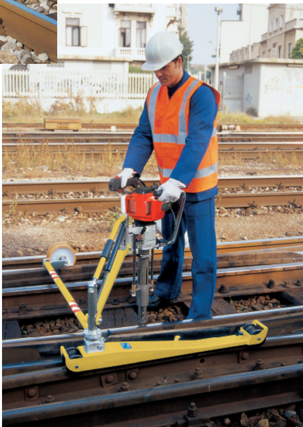
FIG. 6 USING THE DRILLING MACHINE IN CONJUNCTION WITH THE SUPPORT TROLLEY
