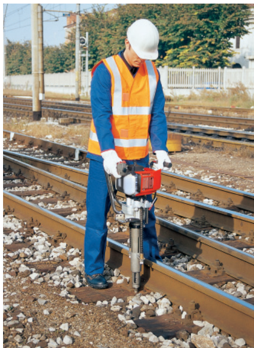
FIG. 5 USING THE DRILLING MACHINE INDEPENDENTLY
